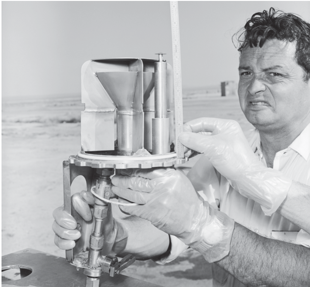
Bill Wilson holds a level sensor and anti-slosh feeder, which were located in each hydrogen-peroxide tank. Baffles prevented pressurized helium from entering the thrusters' transfer lines. (E-14558)
